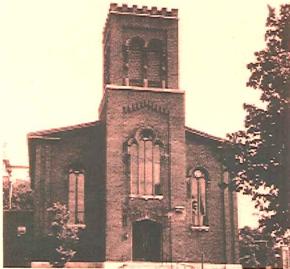
Old Brick, saved
