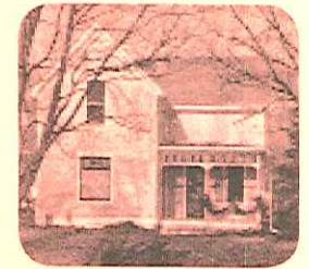
512 Church Street, rehabilitated
