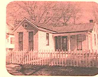
412 Church Street, rehabilitated
